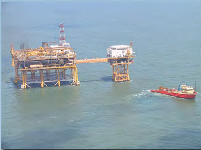
Loop Pumping Platform
